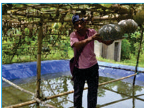
Rainwater harvesting structure (Jalkund)
